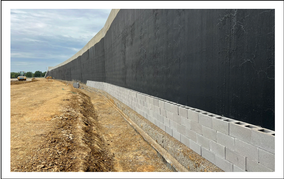
Photo 1 – Installation of back of the wall drainage to Tunnel structure
