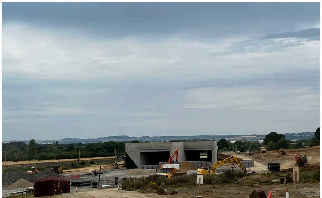
Photo 16 – Southern side of Tunnel – drainage installation
