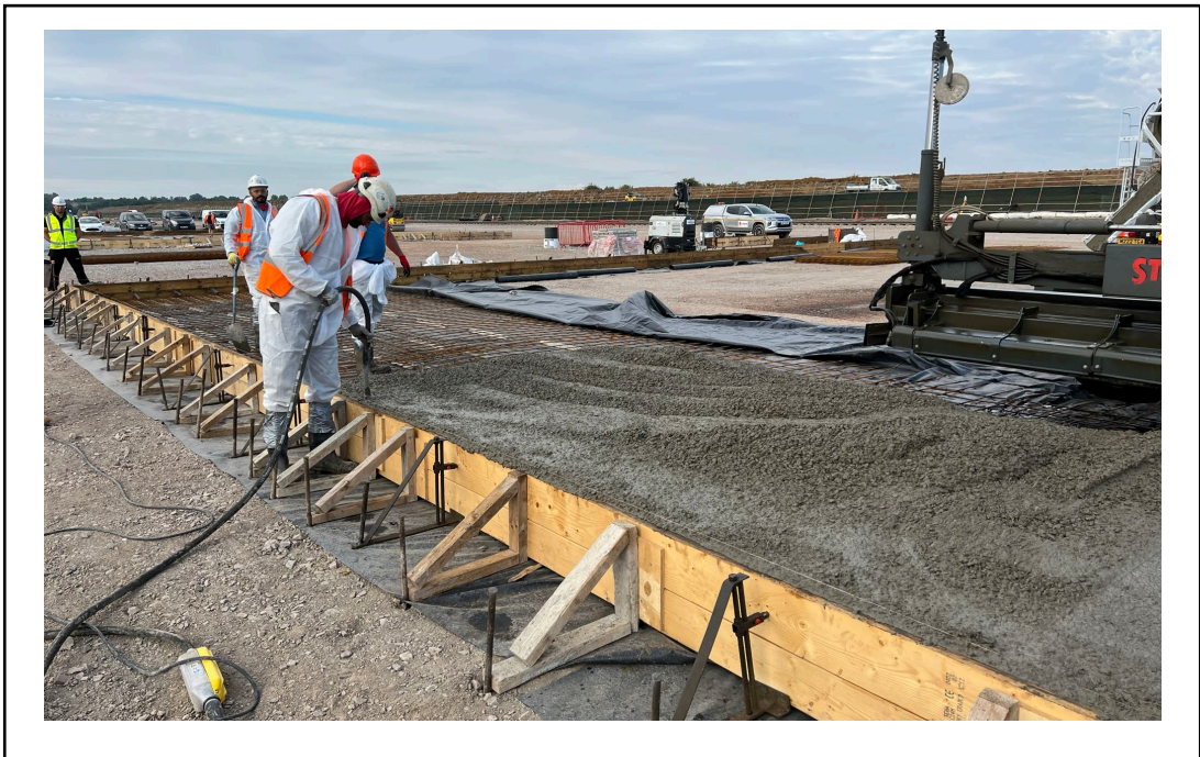
Photo 8 – Terminal concrete slab installation
