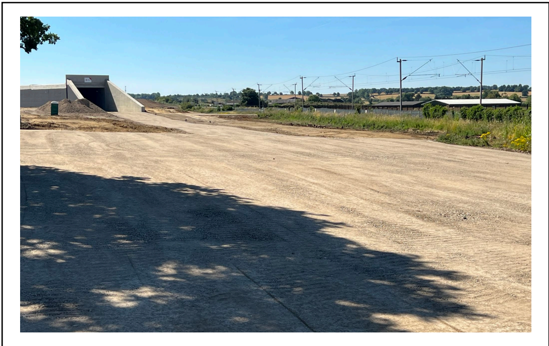
Photo 14 – Northern side of Tunnel structure
