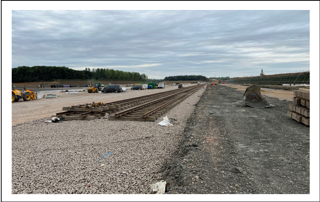
Photo 5 – Rail intermodal sidings view from North to South
