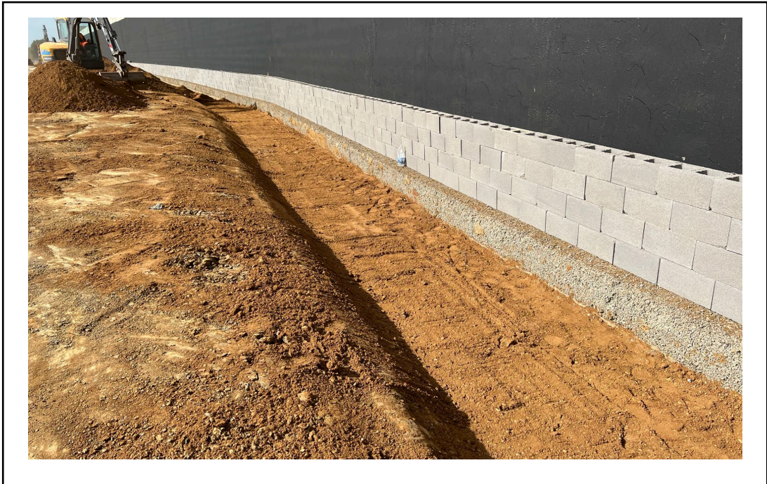
Photo 2 – Bottom layer of the backfill to Tunnel
