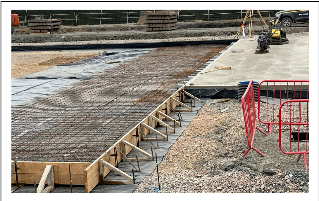
Photo 10 – Terminal concrete slab prep works
