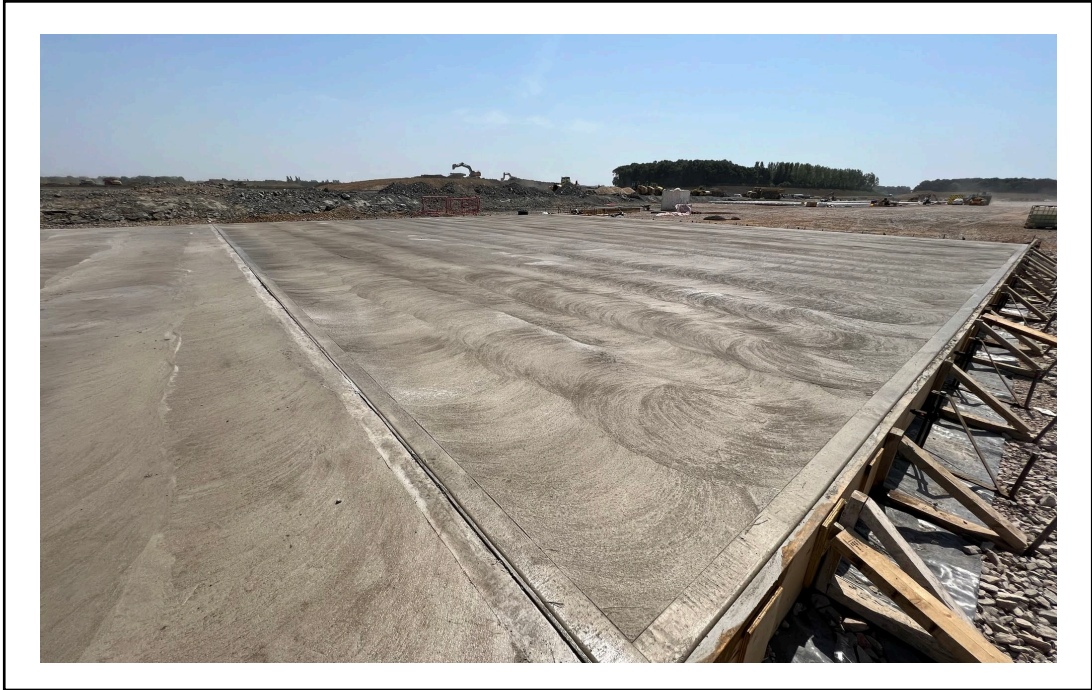
Photo 17 – Northern end of the terminal – slabs
