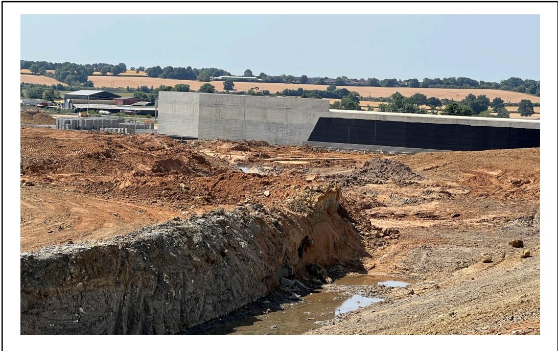
Photo 6 – Earthworks to northern headshunt
