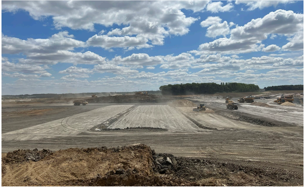
Photo 15 – Earthworks to plot 4
